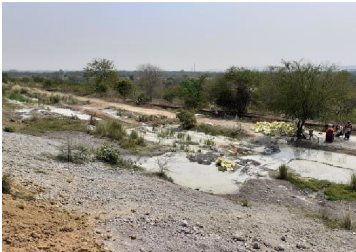
Fig 2. Leakage of fly ash slurry from JPL ash dyke- Photo from Shivpal Bhagat JC Report dated 16.04.2021- page 41
