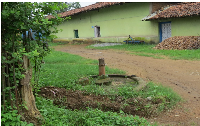
Fig 4. Abandoned hand pump near Gare Pelma IV/2, IV/3 mine in Raigarh, Chhatisgarh. Earlier, these hand pumps had water at hardly 30-40 feet below ground levels, but they had to be abandoned as the water levels fell sharply. (Photo does not necessarily represent current status). Photo Credit: Shripad Dharmadhikary
