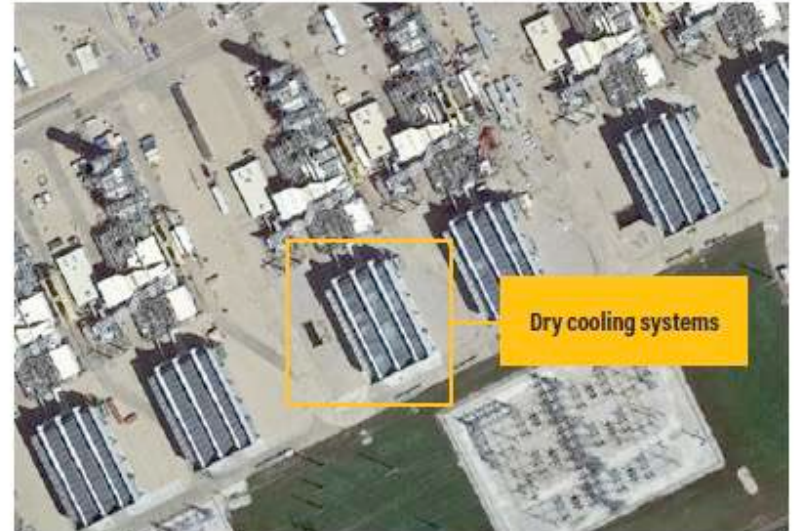
Figure 7 | Satellite Image of a Dry Cooling System
