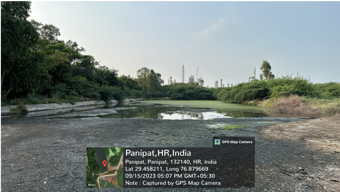
Fig 6: Polishing pond where effluent discharge from the refinery is collected
